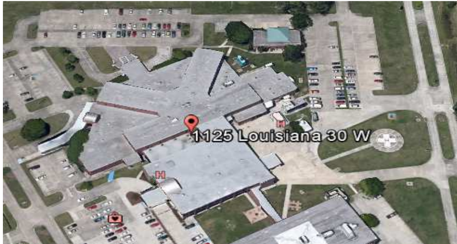
Figure 2. St. Elizabeth Hospital Location
